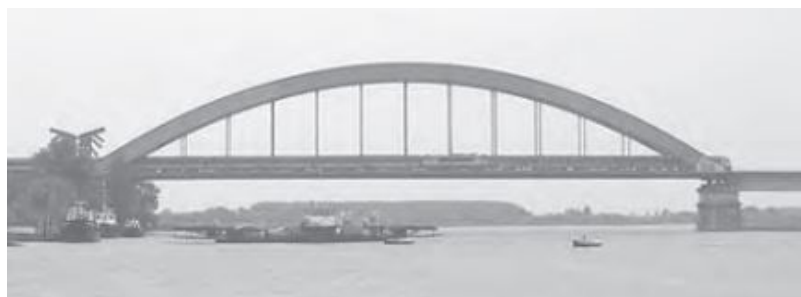
Arches support their loads in compression
