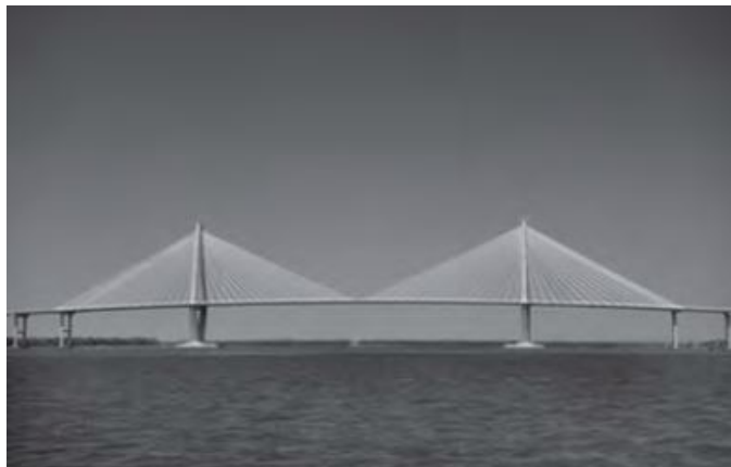
Cables support their loads in tension
