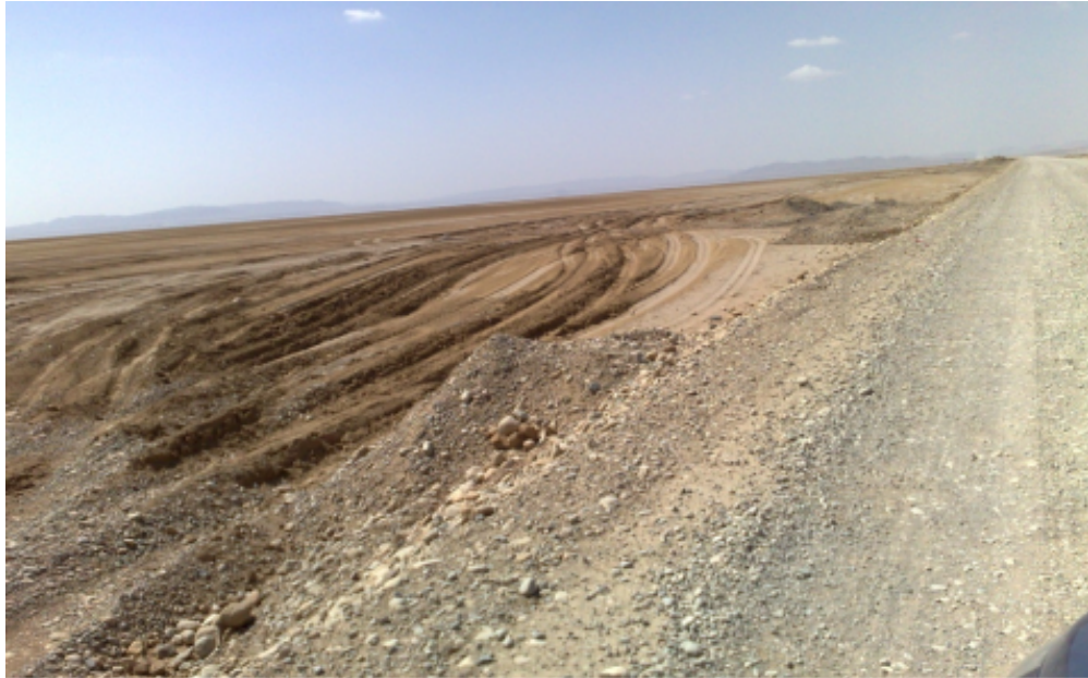
Embankment on compressible soil (Chott El Hodna)
