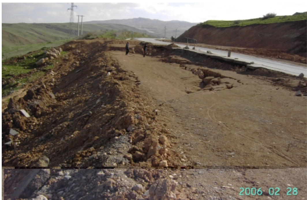
Embankment slide during RN 79A repair works (Mila, 2006)
