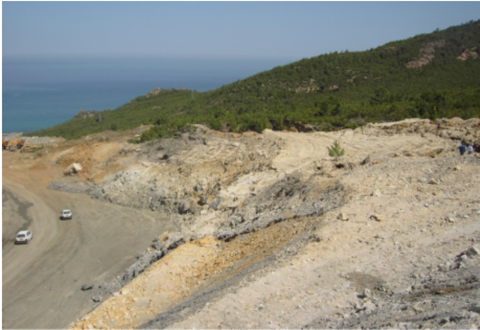
Slide caused by earthworks (Jijel Bypass, 2008)
