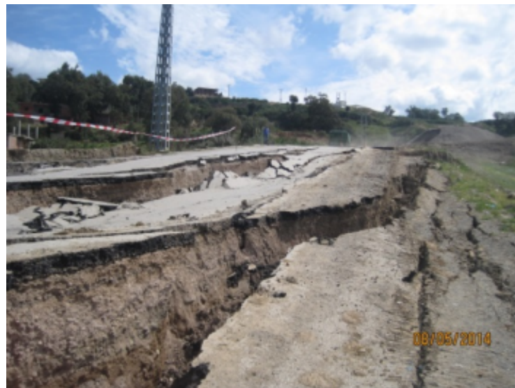
Consequences of exceeding soil shear strength
