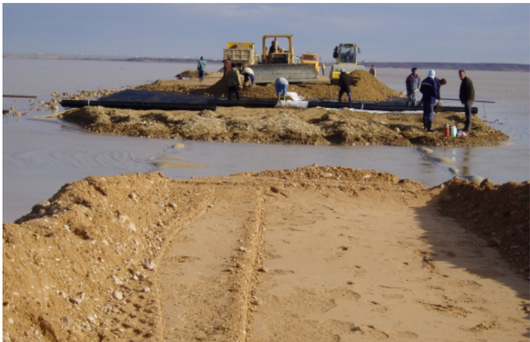
Junction of embankment sections during construction
