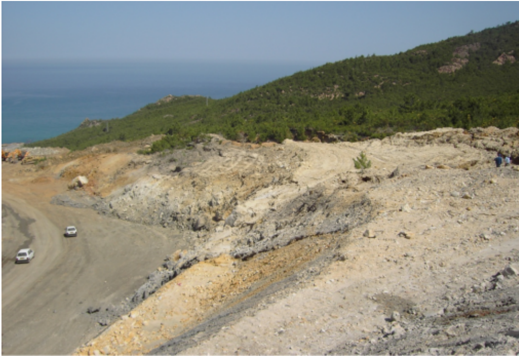
Slide caused by earthworks (Jijel Bypass, 2008)
