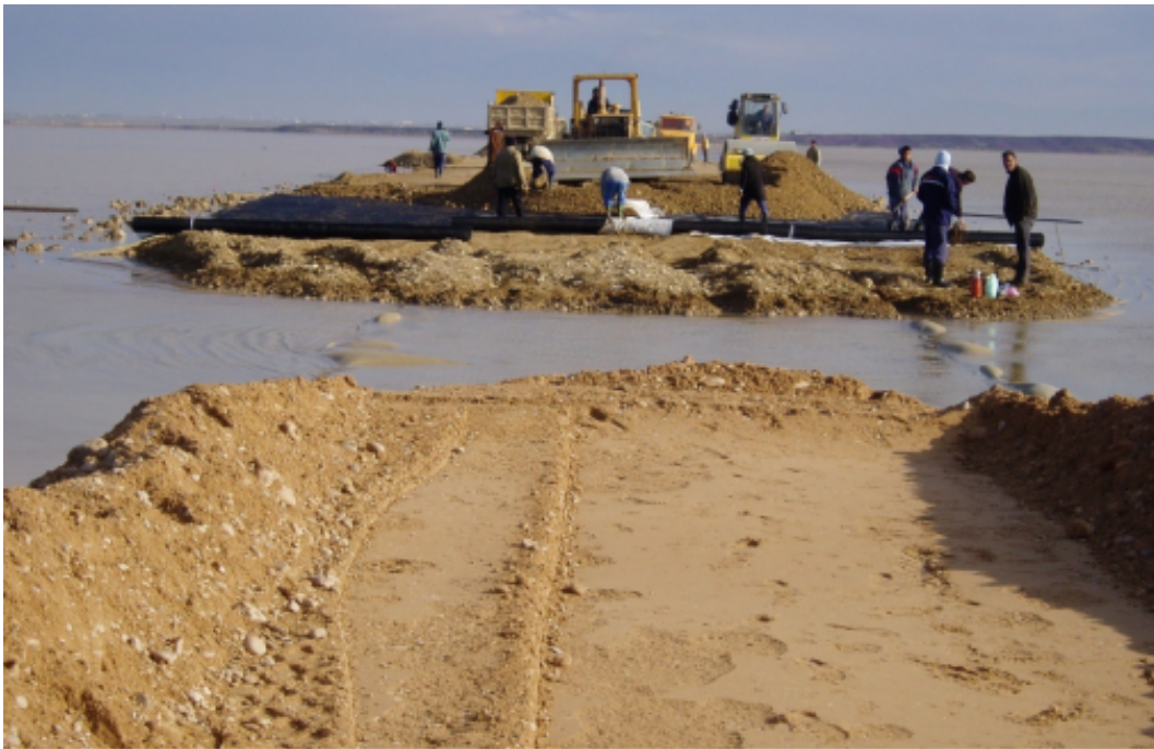
Junction of embankment sections during construction
