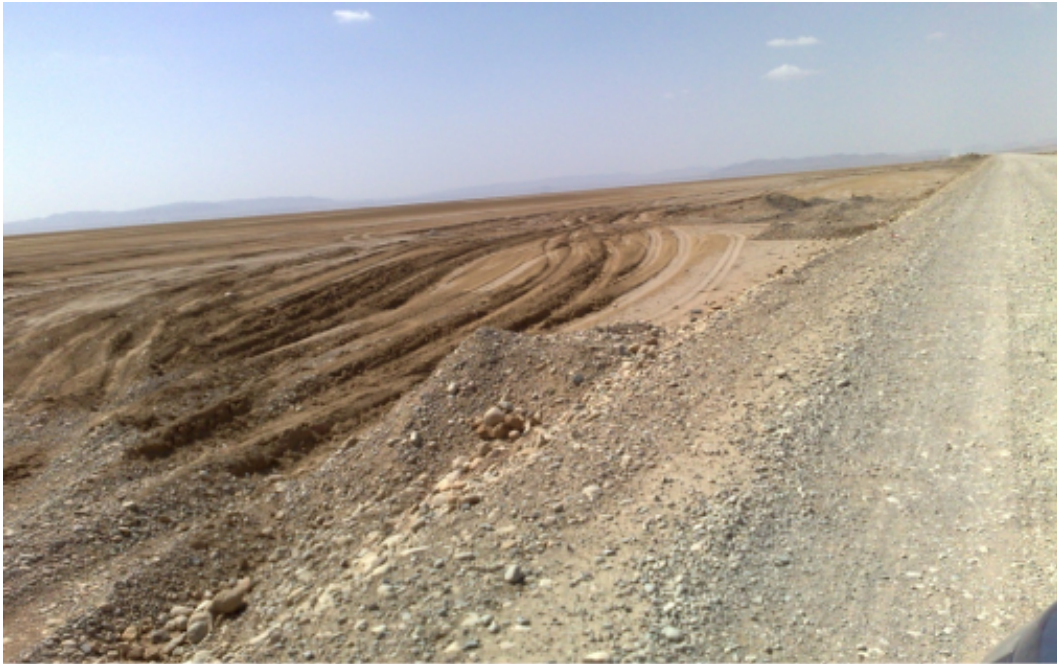
Embankment on compressible soil (Chott El Hodna)
