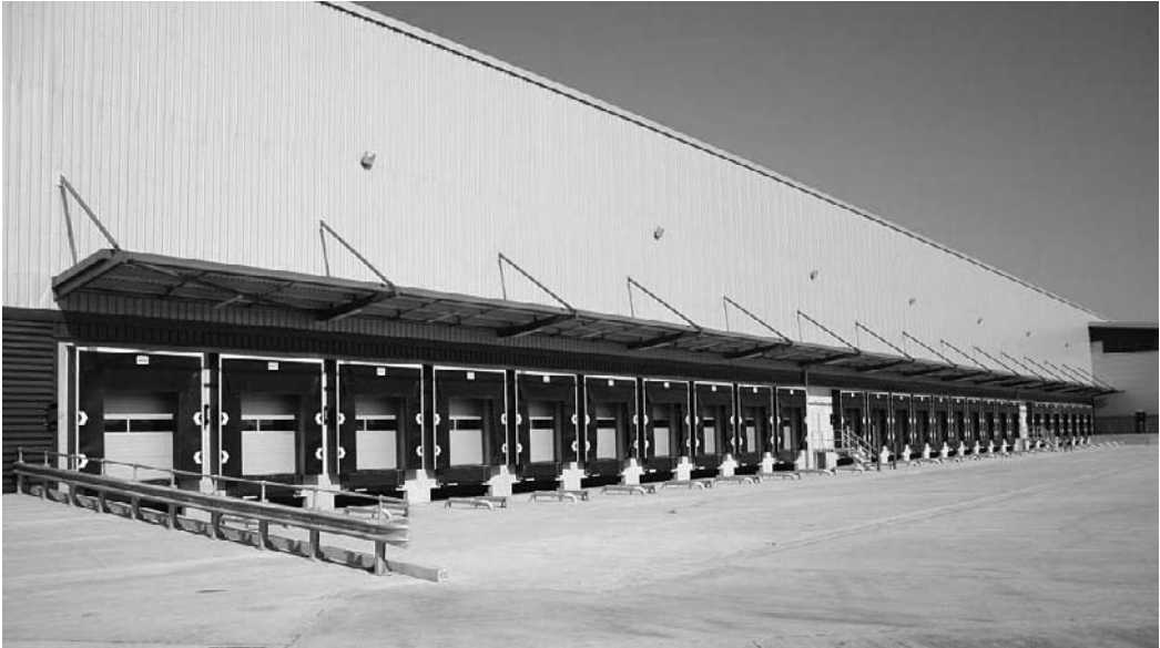
Figure 19.3 Raised dock loading bays (courtesy of Stertil)
