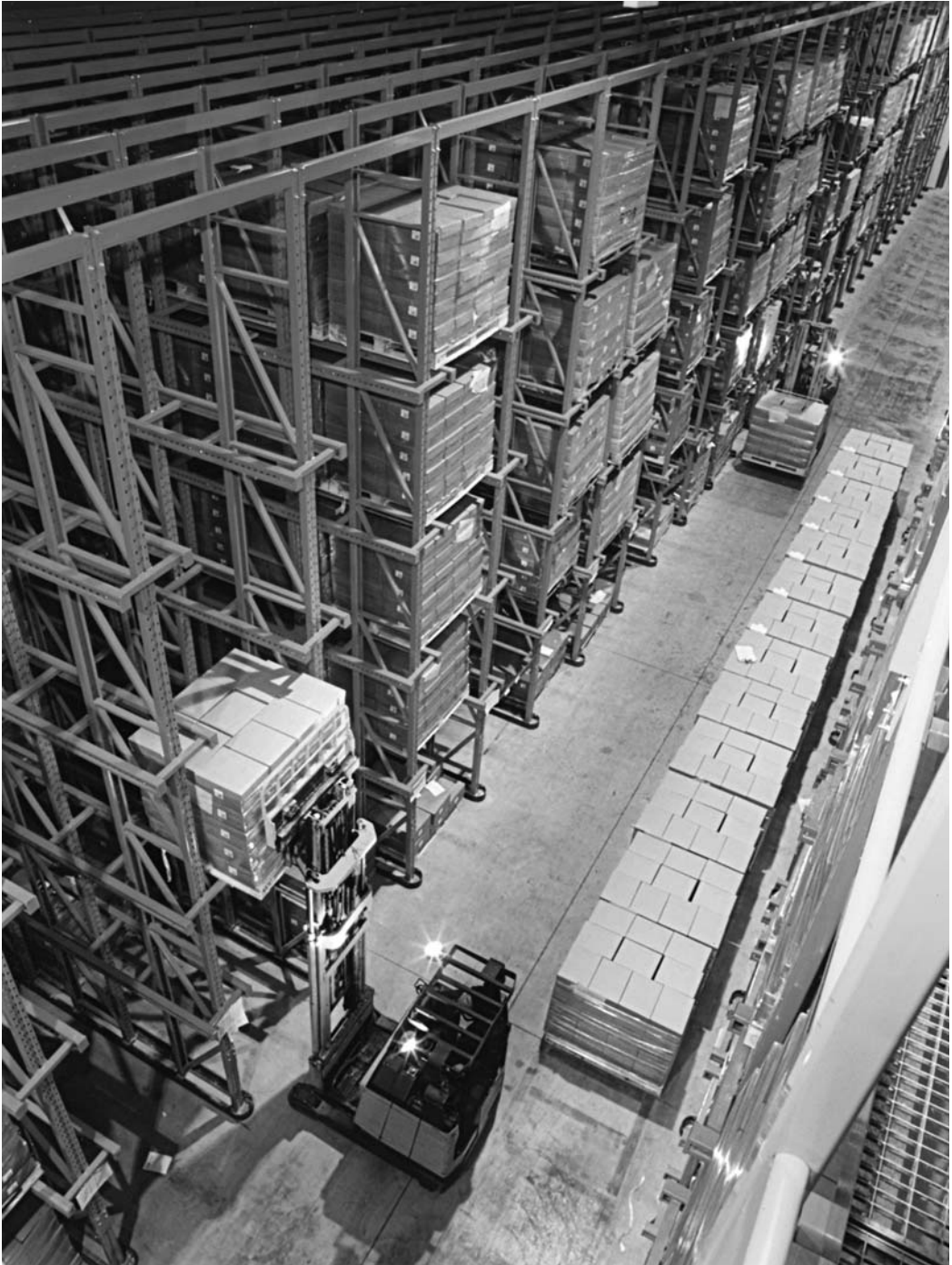
Figure 16.3 Drive-in racking, being served by reach truck (courtesy of Redirack)
