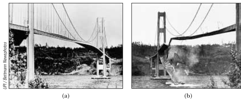
Figure 15.26 (a) In 1940 turbulent winds set up torsional vibrations in the Tacoma Narrows Bridge, causing it to oscillate at a frequency near one of the natural frequencies of the bridge structure. (b) Once established, this resonance condition led to the bridge's collapse.
